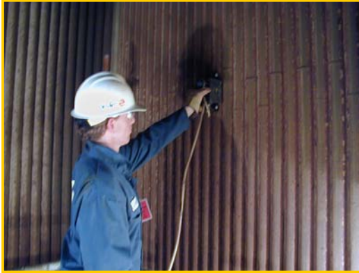
Water wall scanning is being done
