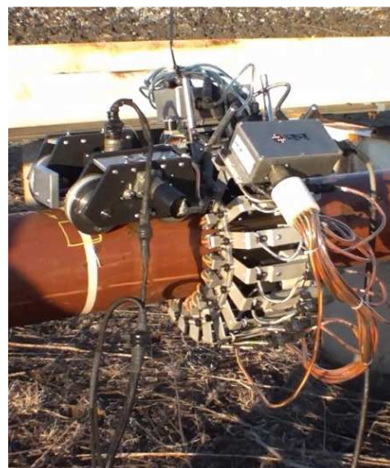
Equipment assembled on the pipeline
